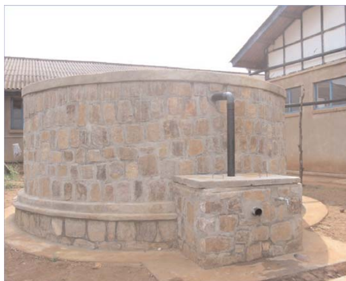
A new cistern for clean water, built through DIF grant.
